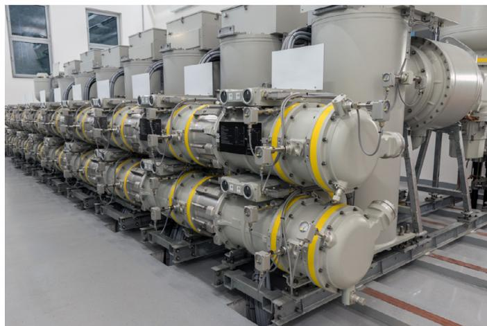
**Figure 1. High-Voltage Gas-Insulated Switchgear (GIS) in Utility Substation.**
